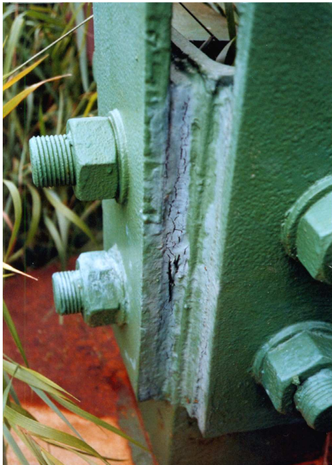
RPCS 10 - cracks in paint and cement
