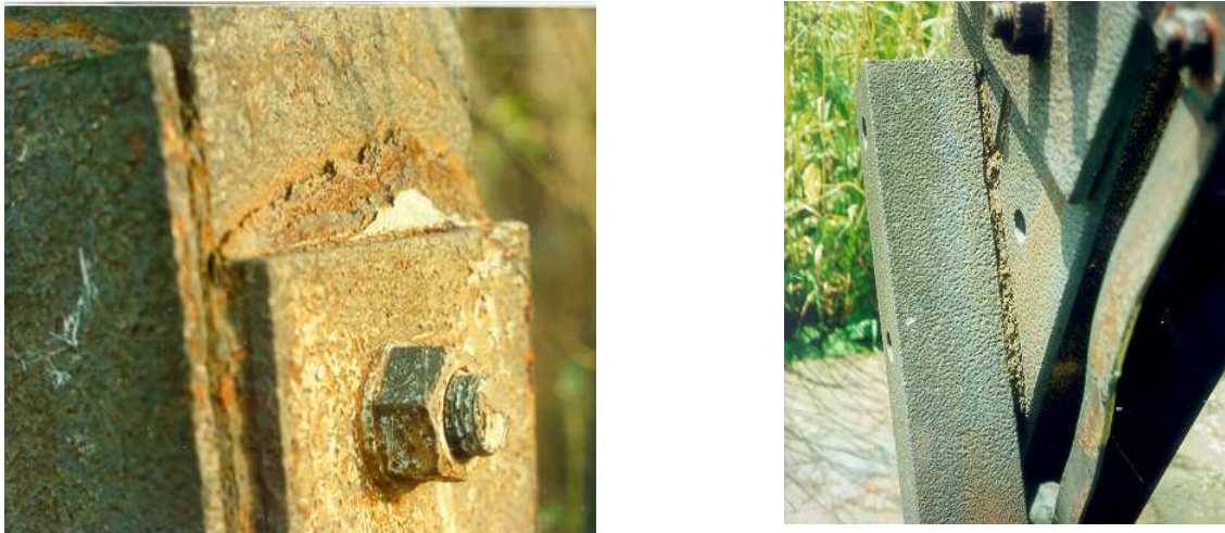
Figure 1 - Typical crevice defect
