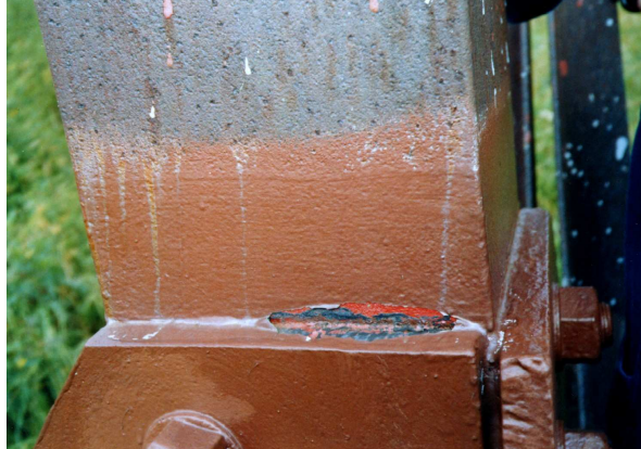
RPCS 10 - big blister in paint and cement
