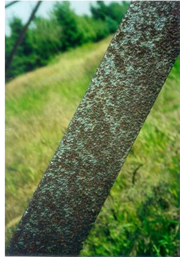
Less protective patina on weathering steel
