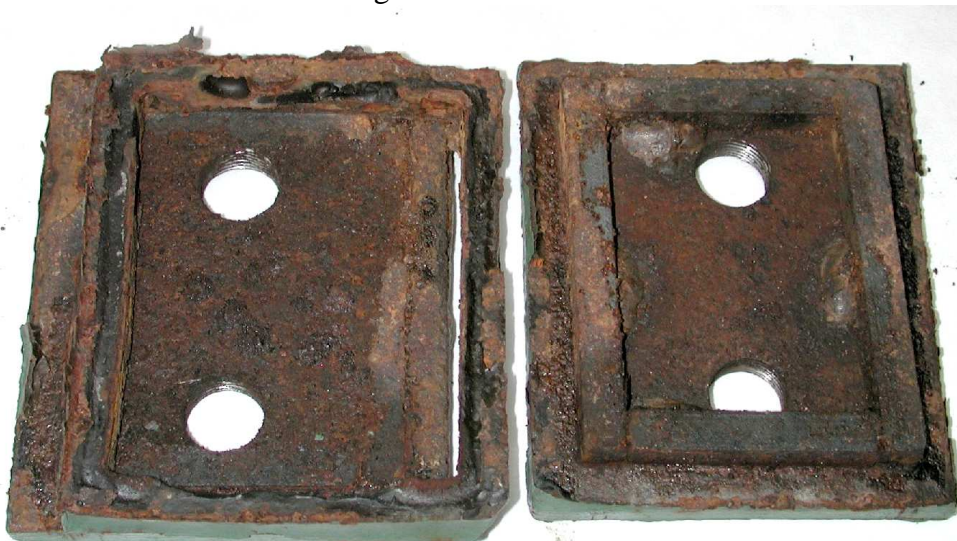
RPCS 11 - Total deterioration of system
