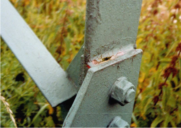
RPCS 10 - total degradation of system
