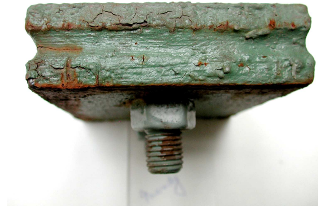
RPCS 11 - total deterioration of system
