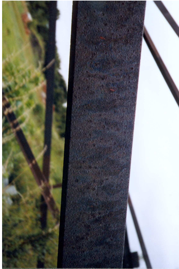
Protective patina on weathering steel
