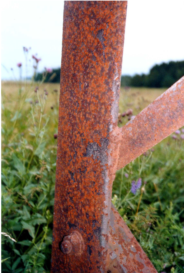
Rust layer on carbon steel
