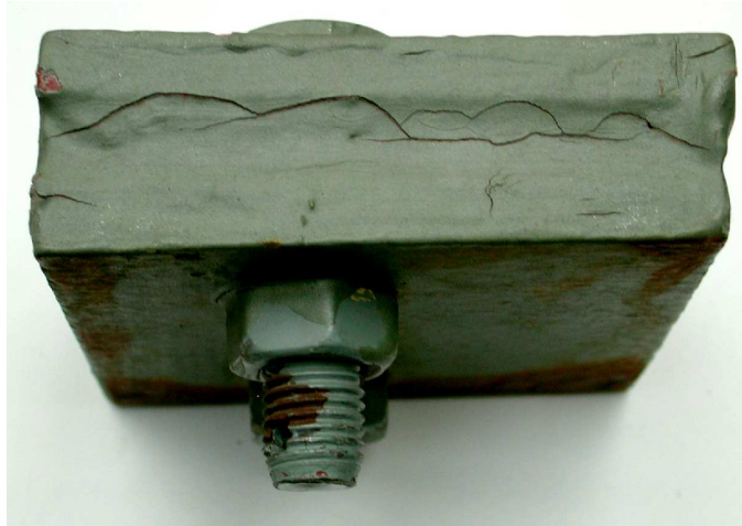
RPCS 1 - cracks in paint
