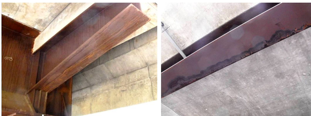
Figure 8 – The negative patina appearance in bridge areas affected by leakage due to non-suitable design and missing gutter after 2 years of exposure
